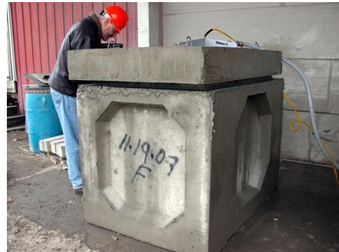
Ron Thornton, Delta Engineers, Binghamton, checks for damage and deflection while the inlet endures H-20 load.
