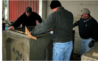
ConSeal on wet concrete seals without sticking.
