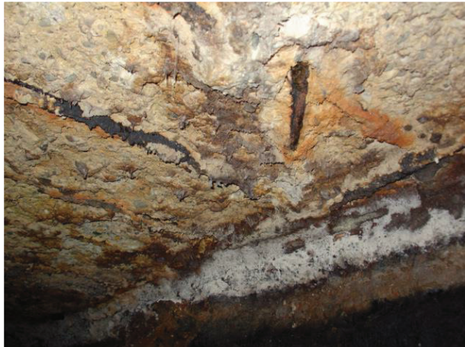
Example of MIC in a wastewater system.
