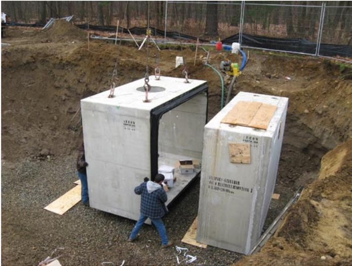
With ConSeal in place the pieces are carefully brought together. The “inside” seal is CS-102. It is seen here on the leading edge of the spigot. The “outer” seal is CS-235 Rapid Expanding Sealant. CS-235 will swell upon contact with water. Extra insurance for water tightness.
