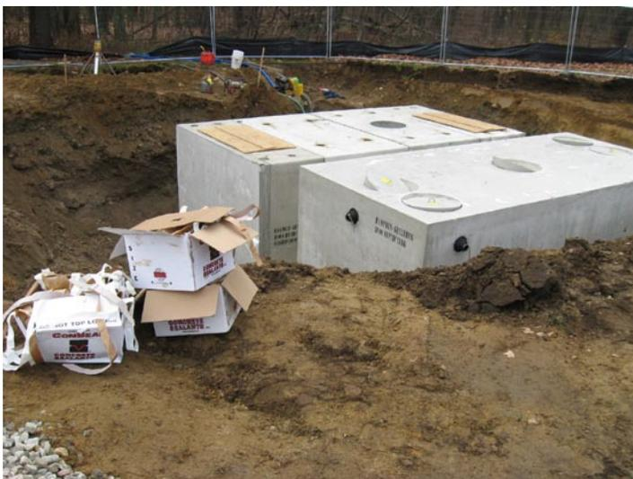
The septic tank is second in a treatment train of three vessels. The first, another 8,000 gallon tank receives the sewage from an elder community. It sends effluent to this tank, which then flows to the recirculating tunnel tank. Septage is pumped to a sand filter which drains back to the second tank. After a number of passes, the treated effluent is dispersed to a drain field.
