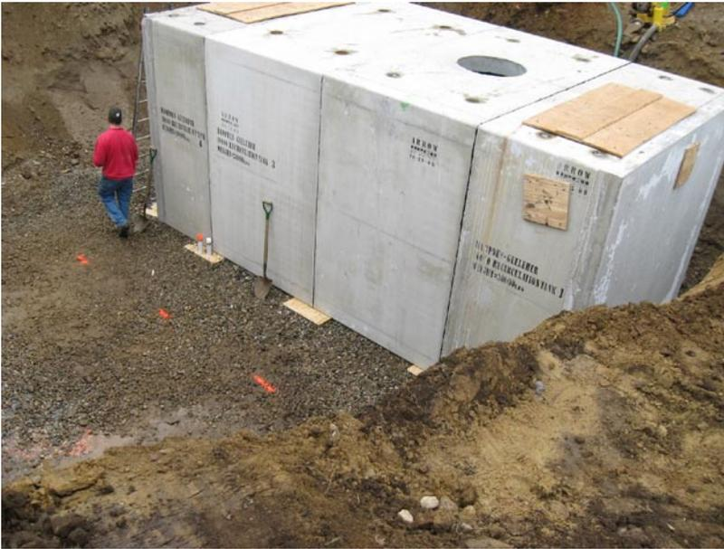
The tunnel tank is a 10,000 gallon recirculation pump tank. It cannot leak! Orange lines on the prepared base indicate where to put an 8,000 gallon septic tank.
