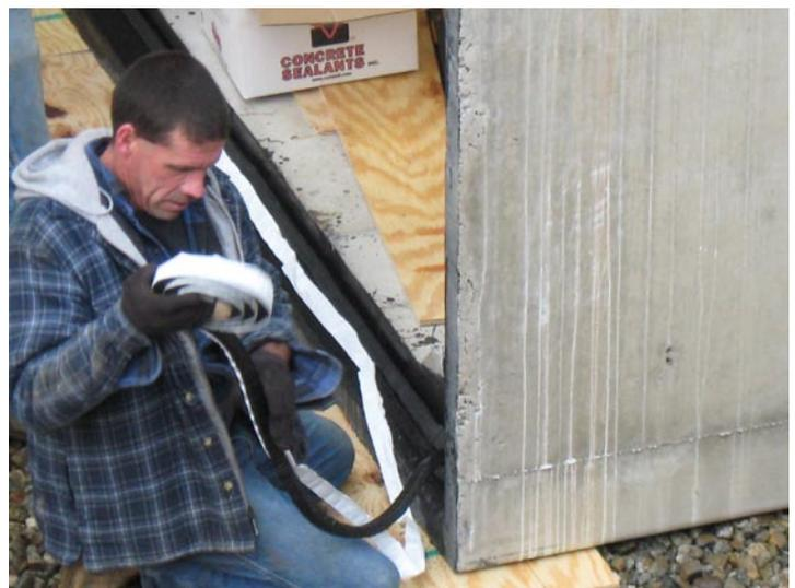
Matt Wench is Product Supervisor for Tunnel Tanks. Today he installs CS-235 Rapid Expanding Sealant
