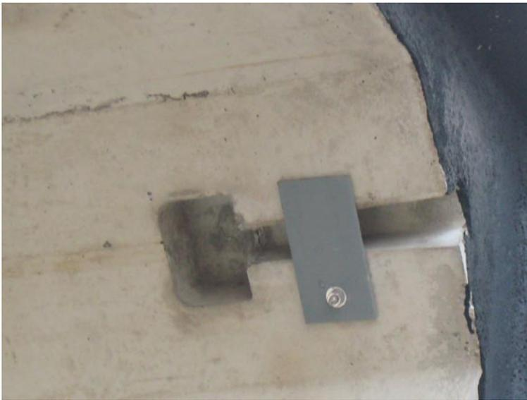
Top bolt pockets are equipped with this guard, which keeps the bolt from dropping on Phil's head while he tightens the bottom bolts.
