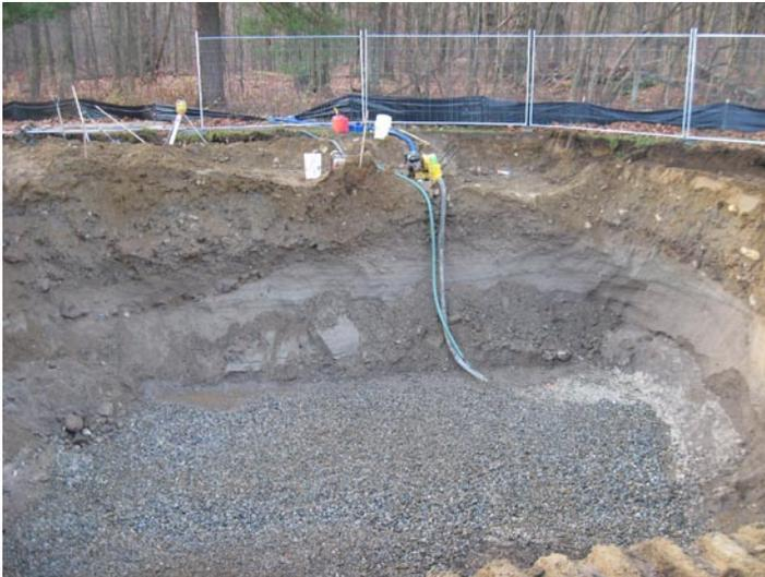
With a pump to relieve groundwater, the level compacted base of 3/4 inch stone is prepared to receive the precast components. Well drained glacial soil is typical to the area.
