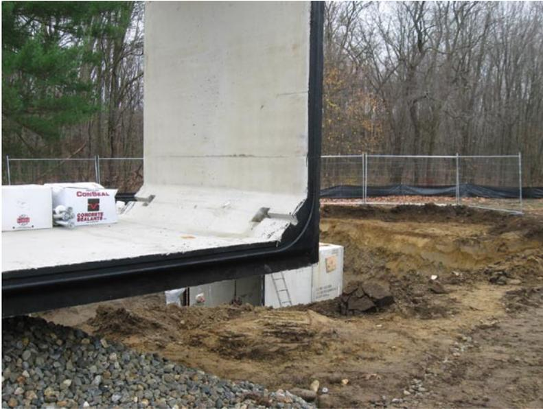
A good view of Bolt Pocket arrangement. This joint was primed in the plant with CS-50 Liquid Rubber Primer. Additional primer and a continuous strip of CS-102 will be applied just before joining the sections.
