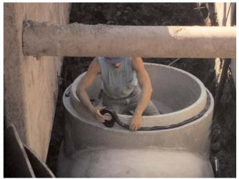
Two strips, one as here, and another on top of the spigot virtually guarantess a water-tight joint.
