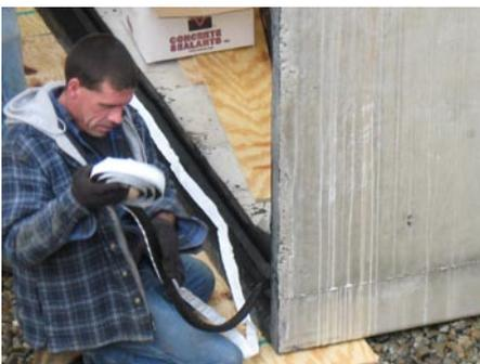
In this case the expanding sealant is placed "outside" the CS-102.
