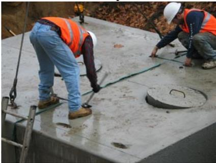
9. Use CS-235 Rapid Expansion water reactive sealant along with CS-102 Butyl gasket.
