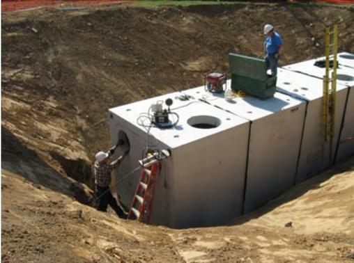
Or use bolt pockets. It seems easier to evenly apply pressure with bolts. Tensioning is usually done with only one power pack which is moved from corner to corner. With tensioning it seems that the boxes "see-saw" their way home.
