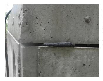
CS-102 is a black butyl gasket. The weight of the concrete compresses it. Some excess butyl "squeezes out" indicating sufficient gasket material is in the joint to make a water tight seal. Neither water nor air ever passes through the gasket. In case of a leak, water sneaks past the gasket, where compression is insufficient. At least 50% compression is the goal.
