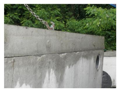
The top slab is poured in a separate adjustable mold. The top of the tank portion is hand finished by one of the workers. The dry fit was pretty good. There were some spots with irregularities, so additional thickness of ConSeal CS-102 butyl gasket was employed to seal the joint.
