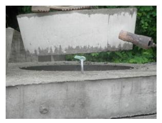
The manhole opening at one end of the tank had to be torch dried. Then it was sprayed with adhesive, which held in place a special gasket from ConSeal, CS-367.
