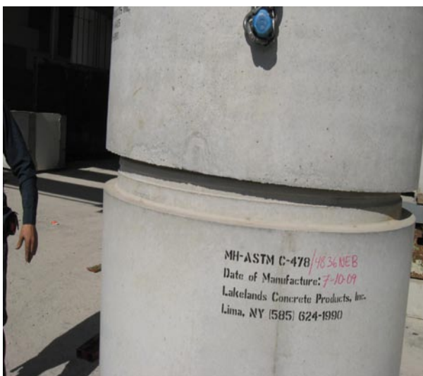
Dry-fit with no gasket material
