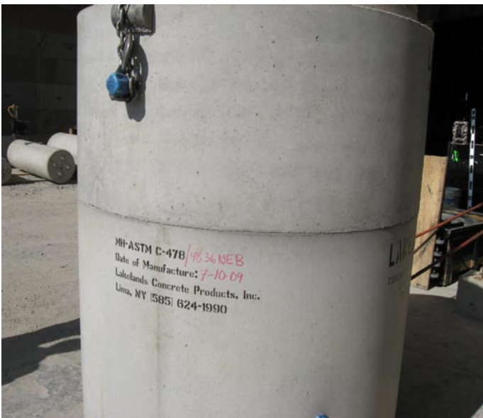
Dry-fit without gaskets. A uniform tight fit
