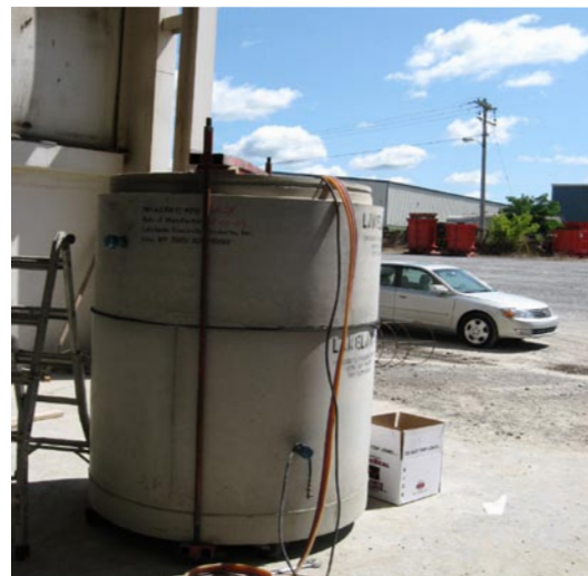
No leaks after 10 minutes= PASS
