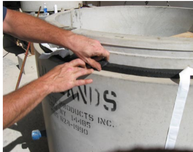
Kneading the ends to make a continuous gasket
