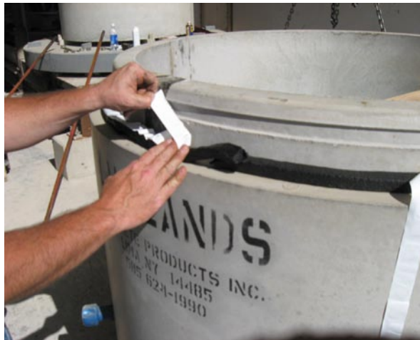
The ends are overlapped, film is removed
