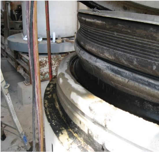
The test ring is positioned to test joint
