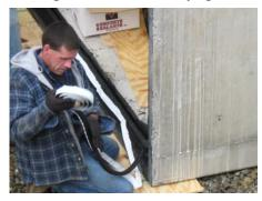
In this case the expanding sealant is placed "outside" the CS-102.
