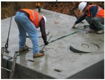
9. Use CS-235 Rapid Expansion water reactive sealant along with CS-102 Butyl gasket.
